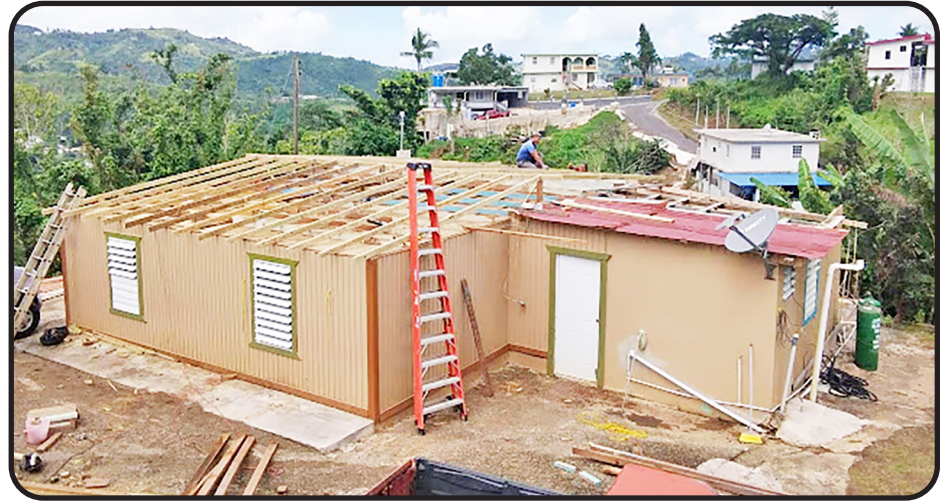
Rebuilding the roof.
