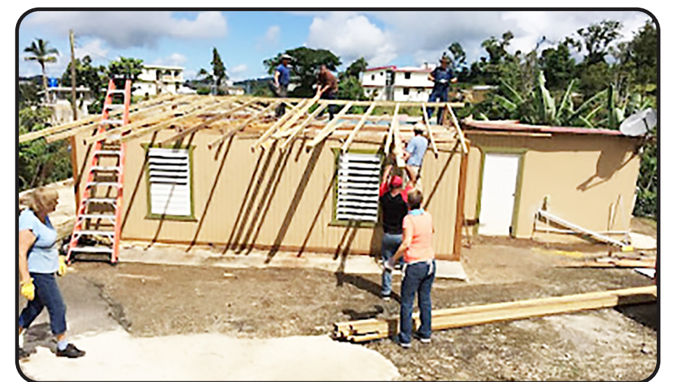
Helping put on a new roof in PR after Hurricane Maria.
