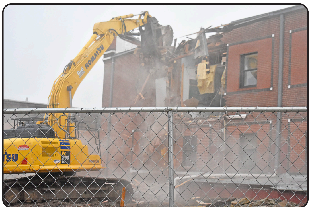
The demolition began
